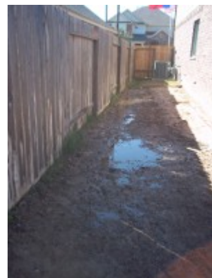
Grading allows pooling near Master bedroom and right side of home.
