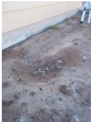
Grading allows pooling near Master bedroom and right side of home.
