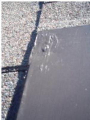
Nail has caulk, but could be better-chimney flashing.
