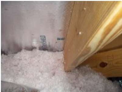
Insulation blocking air movement, but most spaces ave baffle as seen in picture on the right.
