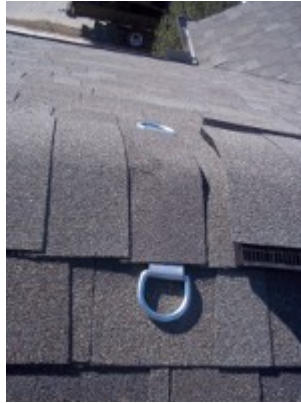
Hook in top roof ridge.
