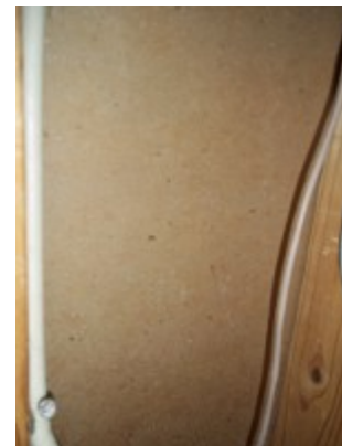
Wiring in return chase.
