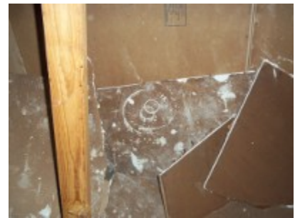
Material left on insulation
