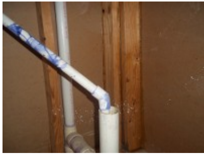
Unsealed return chase. Plumbing in chase is the primary drain for evaporator coil.
