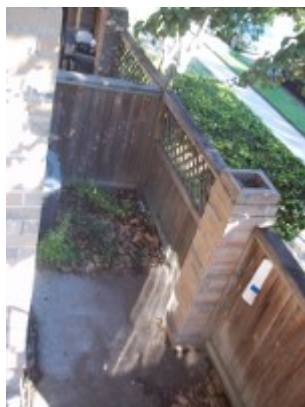
Overview of front porch. Water may pond at the far end due to leaves on the ground.
