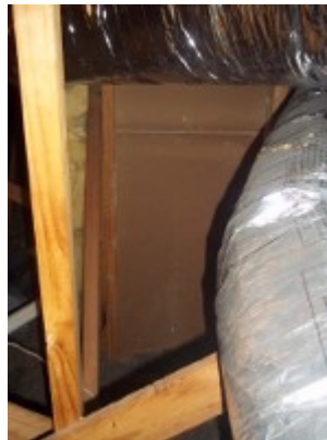
Example of gap in firewall between units.
