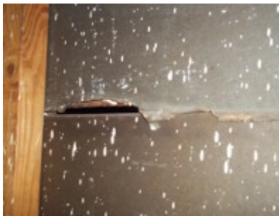
Example of gap in firewall between units.
