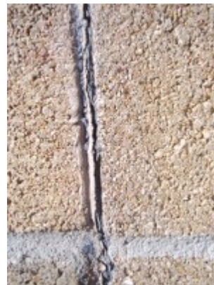
Expansion joint beginning to need new caulking.
