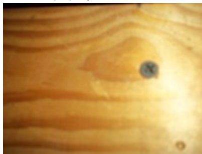
Screw not proper for attic ladder.
